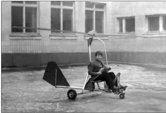
Mr Glushchenko sitting in his autogyro without a powerplant installed.
